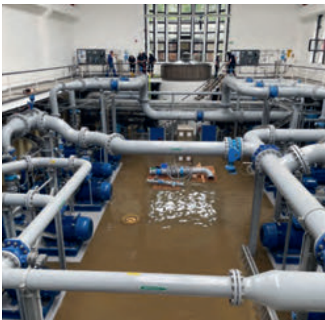
Bild 17.5: Wassereintritt in das Pumpwerk des Wasserwerks Essen-Kettwig (RWW) Fig. 17.5: Inlet of water into the pumping station of the waterworks Essen-Kettwig (RWW)
